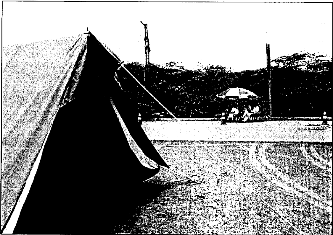
On the site storage arrangement for survey equipment
